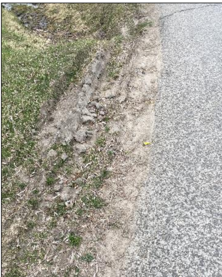
Figure 7: Tire tracks on the shoulder at the northeast corner of the existing truck access and No 2 Side Road location (TNS, 2021).
