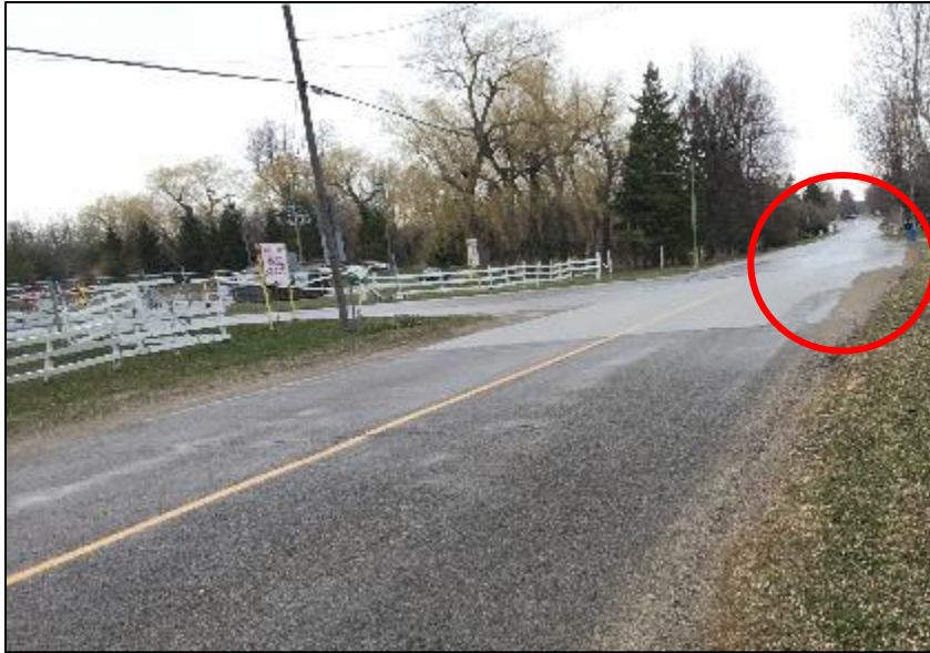
Figure 6: Sand placement showing the path used by trucks turning left onto No 2 Side Road from the existing truck access (TNS, 2021).
